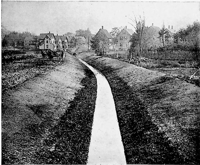
GRAVELLY CREEK LOOKING SOUTH FROM WEBSTER STREET AFTER IMPROVEMENT.
