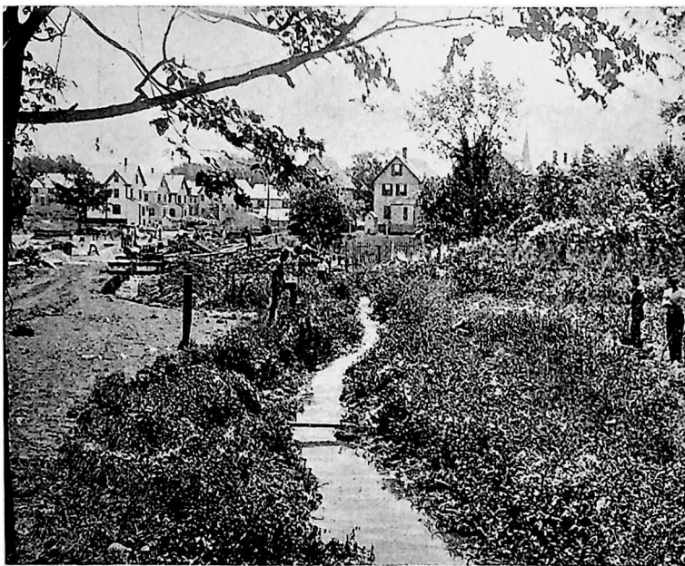
GRAVELLY CREEK LOOKING SOUTH FROM WEBSTER STREET BEFORE IMPROVEMENT.
